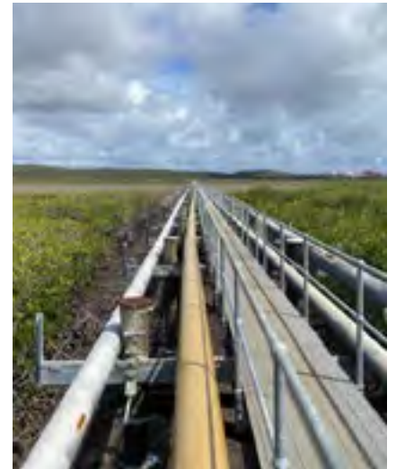
QAL Waste Line Replacement, Australia
