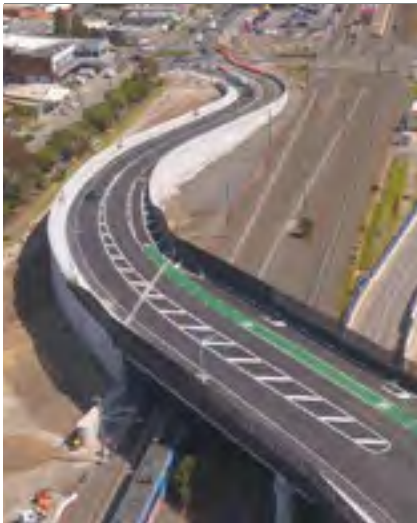
Level Crossing Removal Project, Australia
